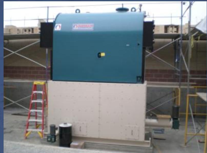
Boiler being installed
