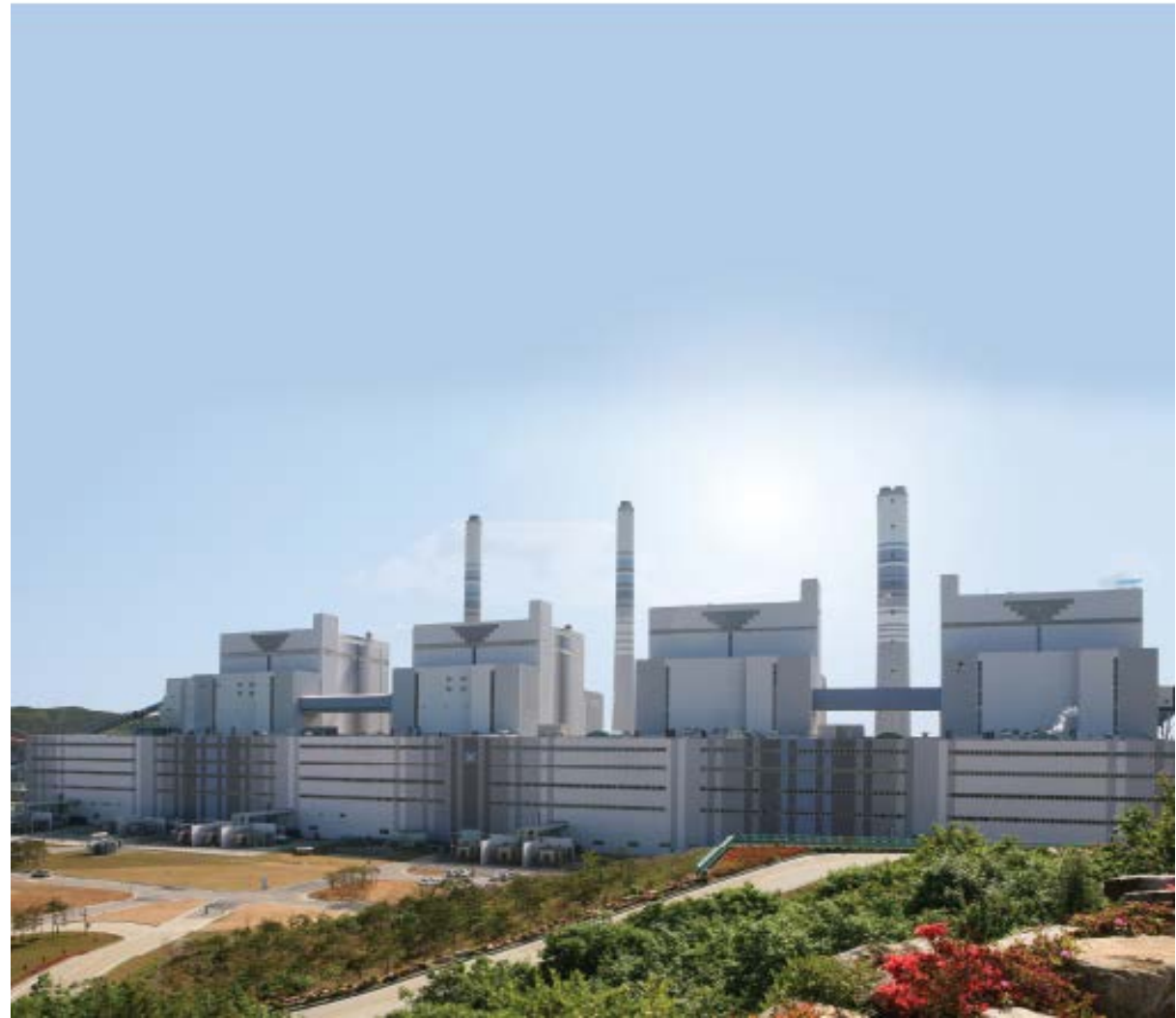
Yeongheung, Korea 5,000 MW Power Station
