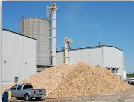
This wood-based 4 MW CHP plant on the Lower Eastern Shore has operated since the 1980s providing heat and electricity to the ECI correctional institution.
