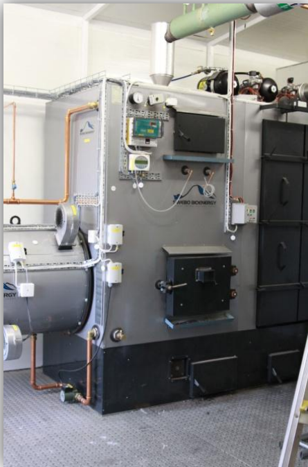
Advanced European wood combustion technology. This 500kW (1.7 MMBtu/hr) biomass boiler produces minimal particulate emissions (0.01 lbs/MMBTU) and operates with an efficiency of nearly 90%.
