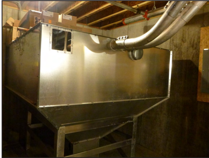
Figure 3: Indoor pellet storage bin with pipes
